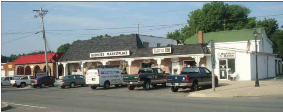
Figure 8 Photographs of Commercial Buildings in the Core District
