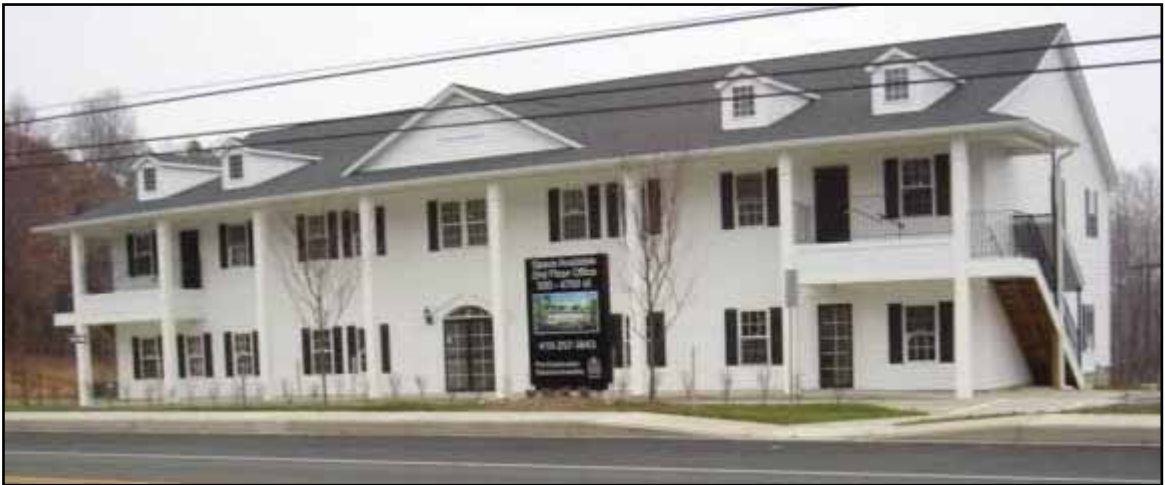
Figure 11 Photograph of Commercial Building in Mixed Use District
