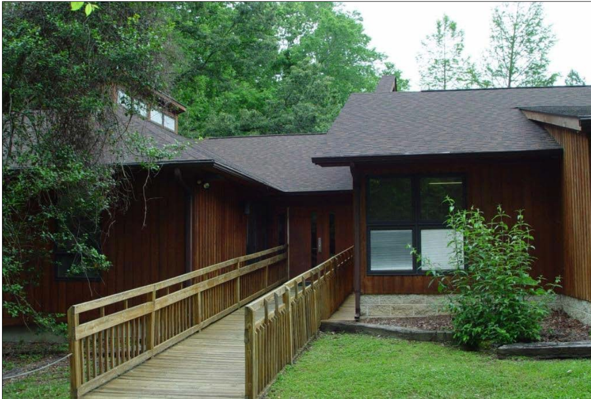
Exterior of building for potential expansion
