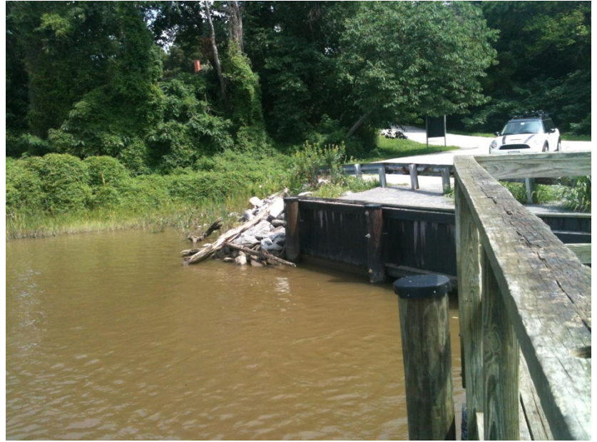
Lower Marlboro Wharf could be renovated to include a kayak/canoe launch.
