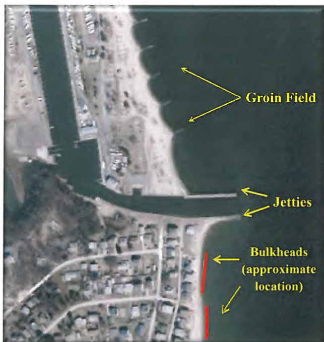
Figure 18: Groin Field & Bulkheads in the Breezy Point and Neeld Estate
