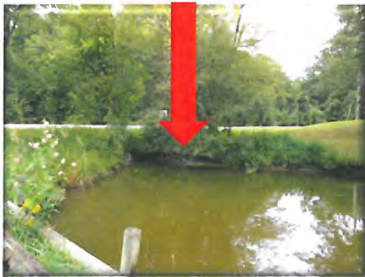
Photograph 5: SHA Nan's Cove Storm Drain, July 31, 2014
