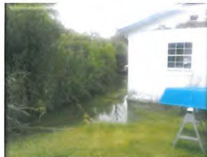
Photograph 3: 2014–Ballard Rogers Road DPW Culvert Stormwater Conveyance Area Flooded
