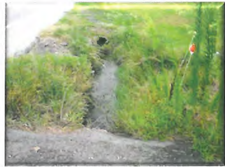
Photograph 6: SHA Culvert – North of Oyster House Road
